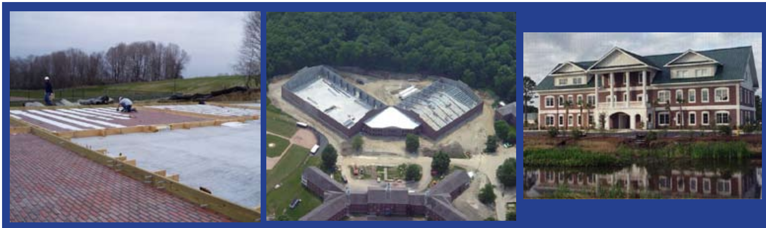
Thin brick allows tilt-up to "adapt" to existing structures.
