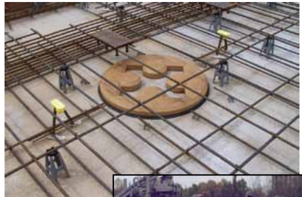
Rebar mat for tilt up project
