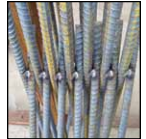
High quality welding
