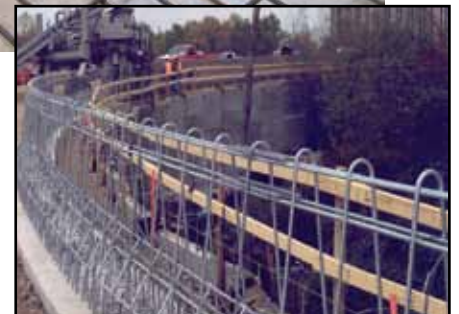
Slipforming Barrier Wall
